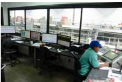
Control room overlooking the fruit sorting chutes.
