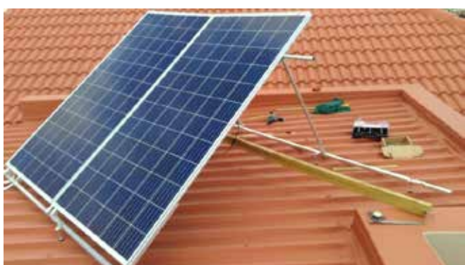
Figure 6. A domestic 650 W PV array.
